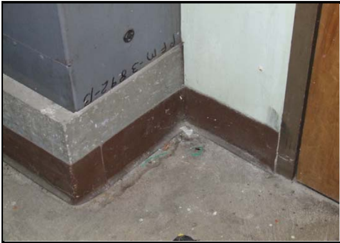
Photo 3 : Brown vinyl cove base HVAC/Boiler Room
