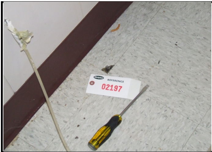
Photo 3 : 12"x12" Gray Tile - Not Asbestos Black Mastic Under Tile 2% Chrysotile Asbestos
