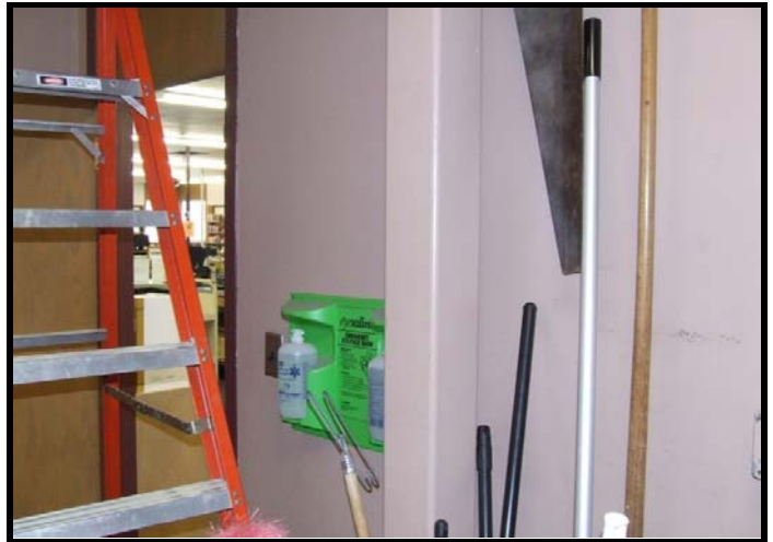
Photo 4 : Beige paint on vertical support beam Janitor's Closet, East wall
