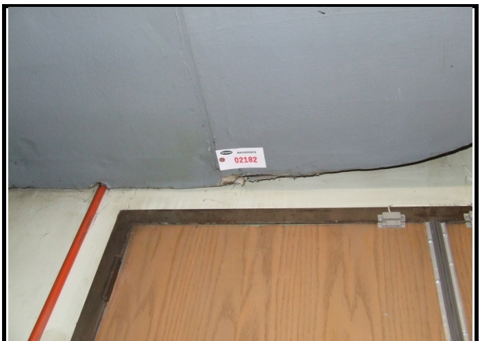
Photo 6 : Non-asbestos Duct Insulation HVAC/Boiler Room
