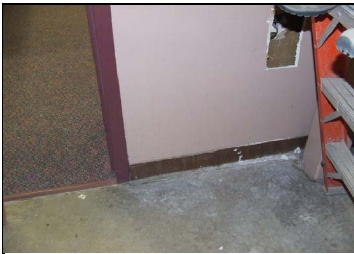
Photo 5 : Brown vinyl cove base Janitor's Closet
